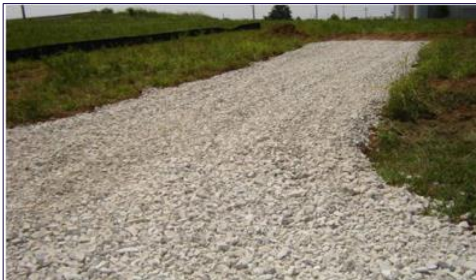
Figure 8.1: Temporary access track
